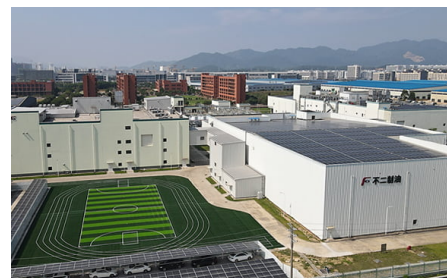
PV panels installed at Fuji Oil (Zhaoqing) Co., Ltd. (China)
