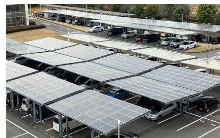
The solar panels installed on carports for the first time at Fuji Oil Co., Ltd.'s Kanto Plant
