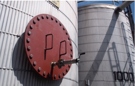
Valve installed on the tank
