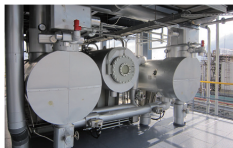
New energy-saving vacuum system for deodorization tower installed at the Hannan Business Operations Complex
