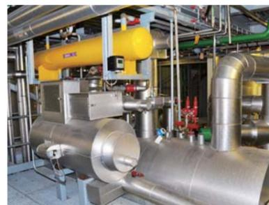
Ice condenser-type vacuum generating apparatus
