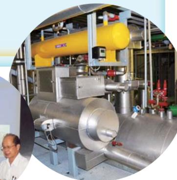
Ice condenser-type vacuum generating apparatus
